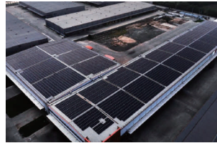
AIKO efficiently utilizes idle rooftops in the industrial park for photovoltaic system installation
