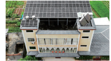
AIKO assists Xinxiang Hotel in Meizhou, Guangdong with its photovoltaic project renovation
