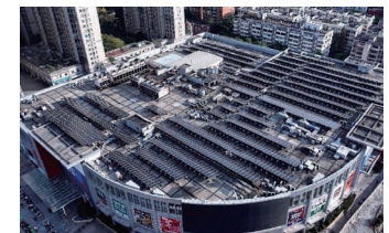
AIKO supports the photovoltaic renovation project of CapitaLand Mall
